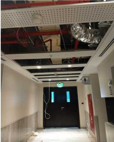
DOHA BANK CORNICHE BRANCH
